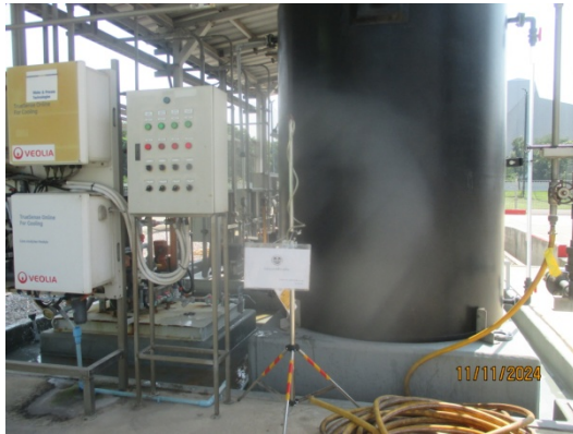
Chemical Feed Cooling Tower Block 1
